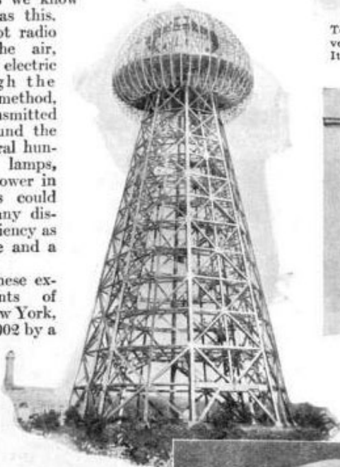
Above: The 200-foot "Tesla's tower" at Shoreham, Long Island, destroyed by dynamite blast in 1914. Its purpose, Tesla explains, was to feed tremendous electric currents into the earth for transmission. At the right is shown the induction motor, one of Tesla's greatest discoveries.
