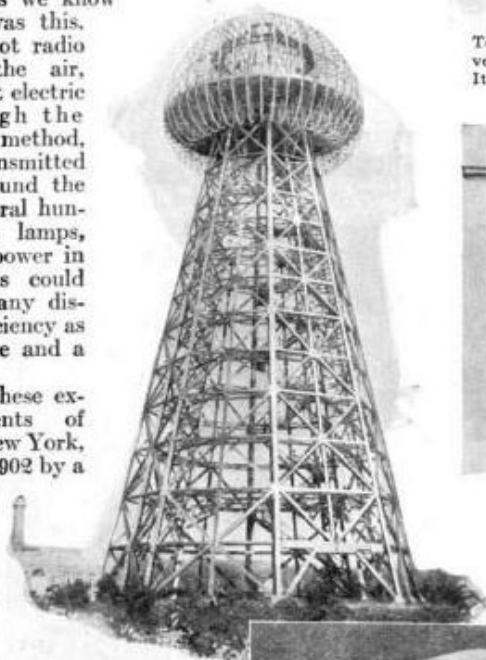
Above: The 200-foot "Tesla's tower" at Shoreham, Long Island, destroyed by dynamite blast in 1914. Its purpose, Tesla explains, was to feed tremendous electric currents into the earth for transmission. At the right is shown the induction motor, one of Tesla's greatest discoveries.
